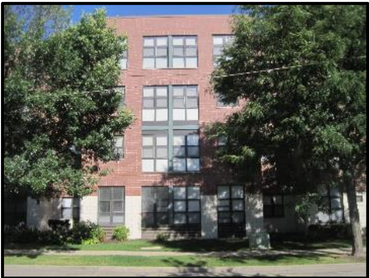
Looking East across the Subject Site
