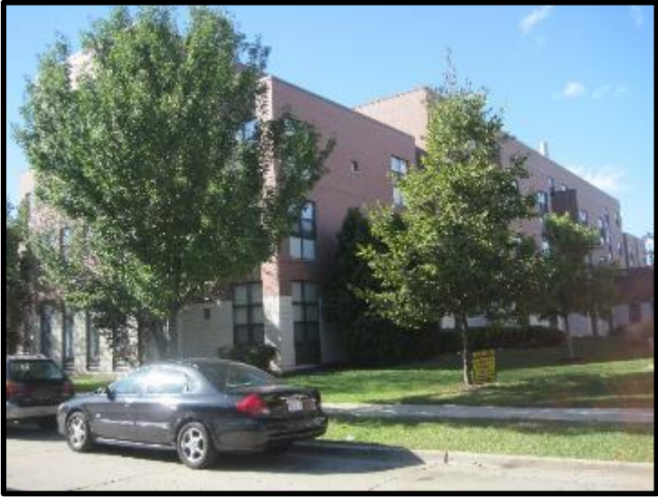
Looking Northwest across 2nd of two Resident Buildings
