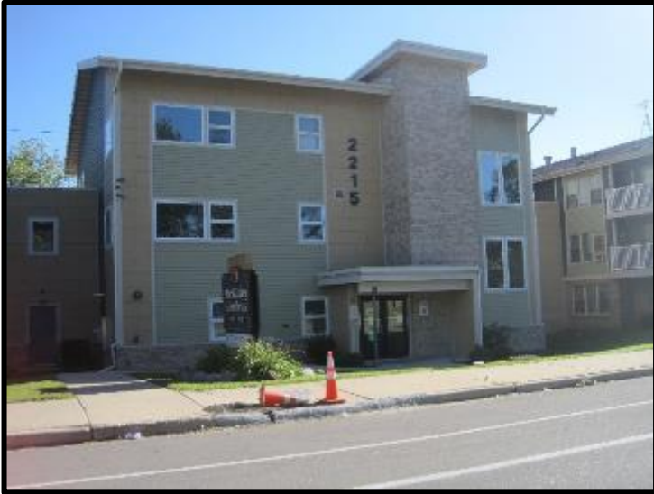
McKinley Gardens Apartments Northwest of the Site
