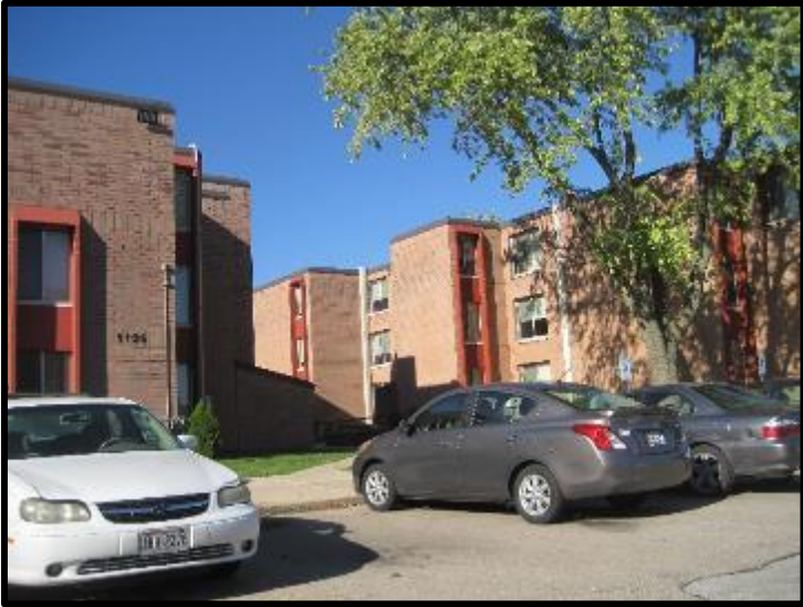
Highland Park Apartments Southeast of the Site
