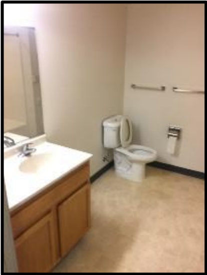
Typical Bathroom in a Unit
