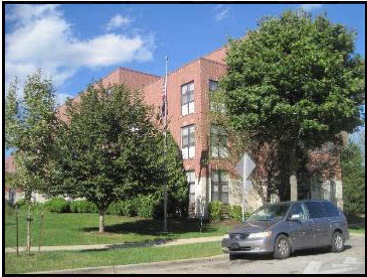
Looking Northeast across one of two Resident Buildings
