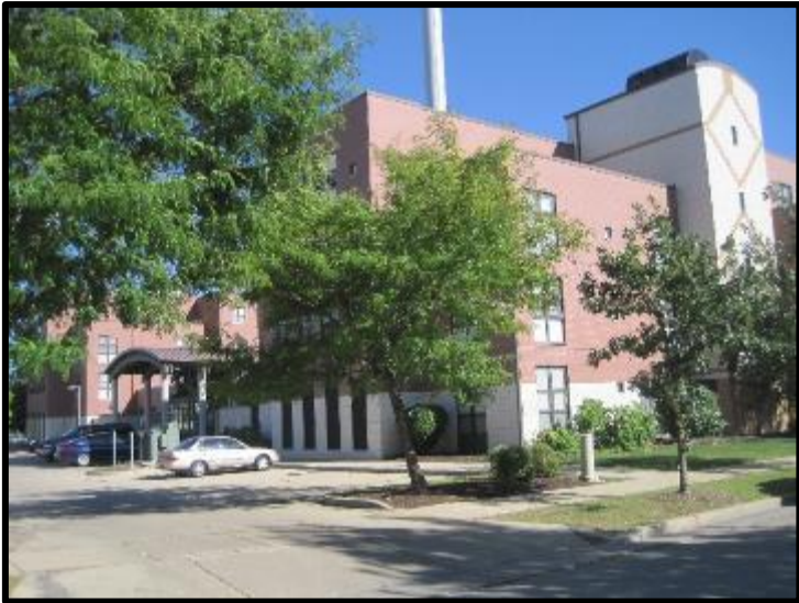
Looking Southeast across the Subject Site
