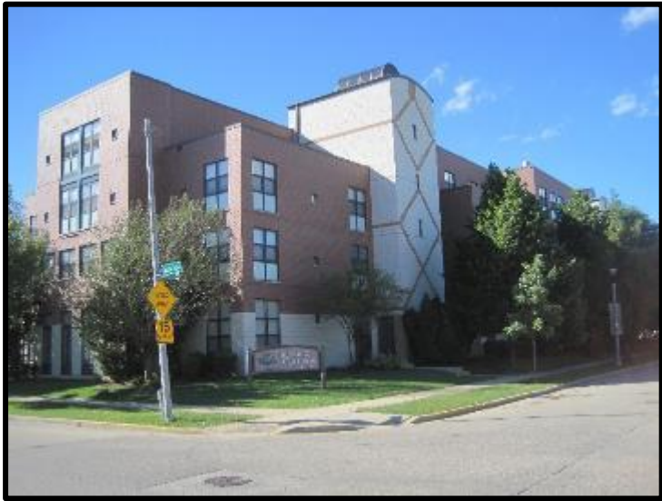
Looking Northwest across the Subject Site
