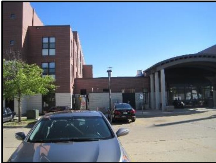
Looking South across the Subject Site
