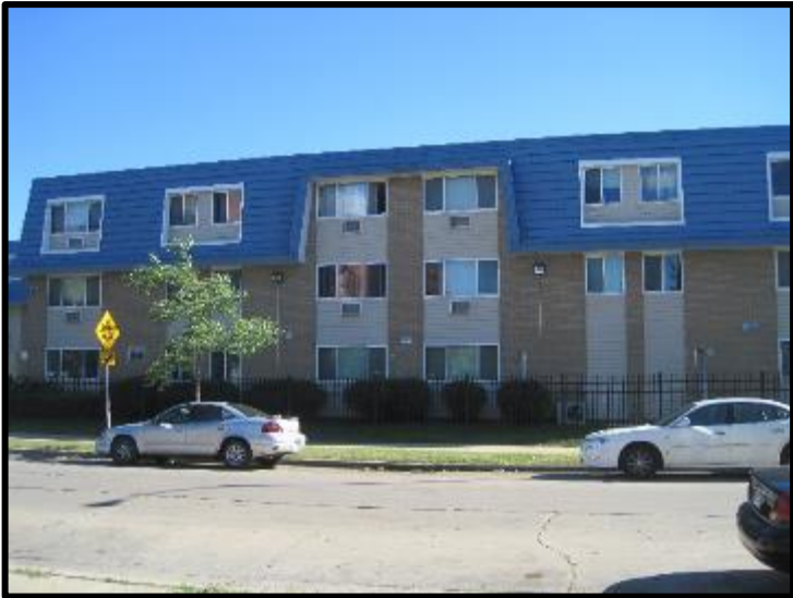
Looking South at the Windsor Court Development from the Subject Site
