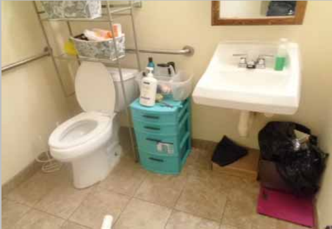
View of typical ground floor / accessible dwelling unit kitchen bathroom.
