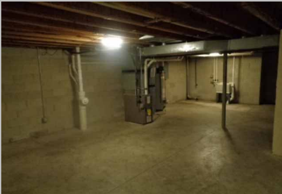
View of typical dwelling unit basement.
