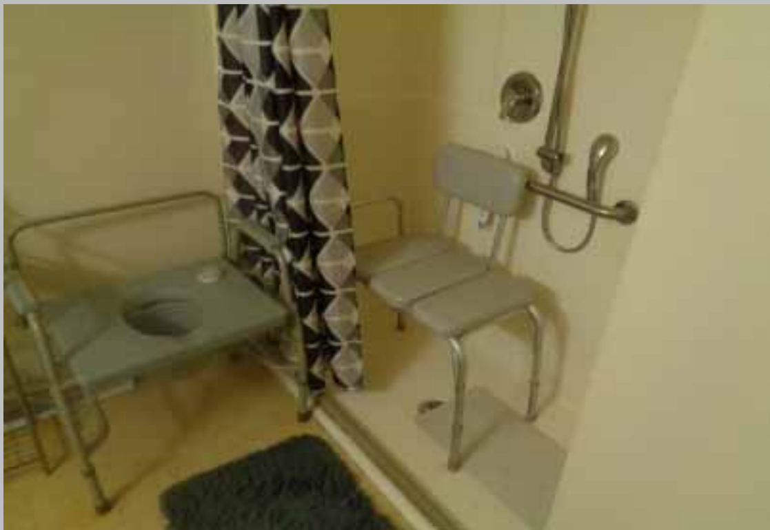
View of typical ground floor / accessible dwelling unit shower.
