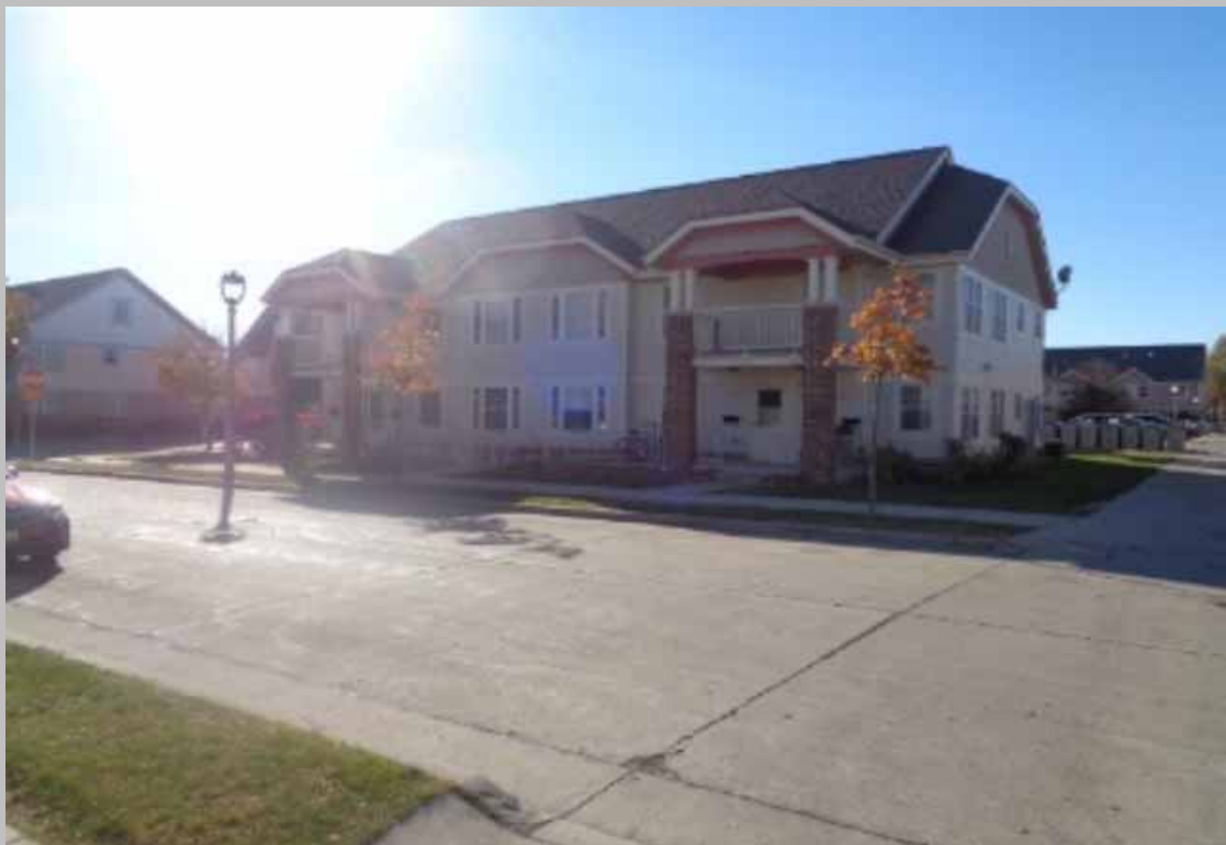
Additional view of typical concrete driveway and parking areas.
