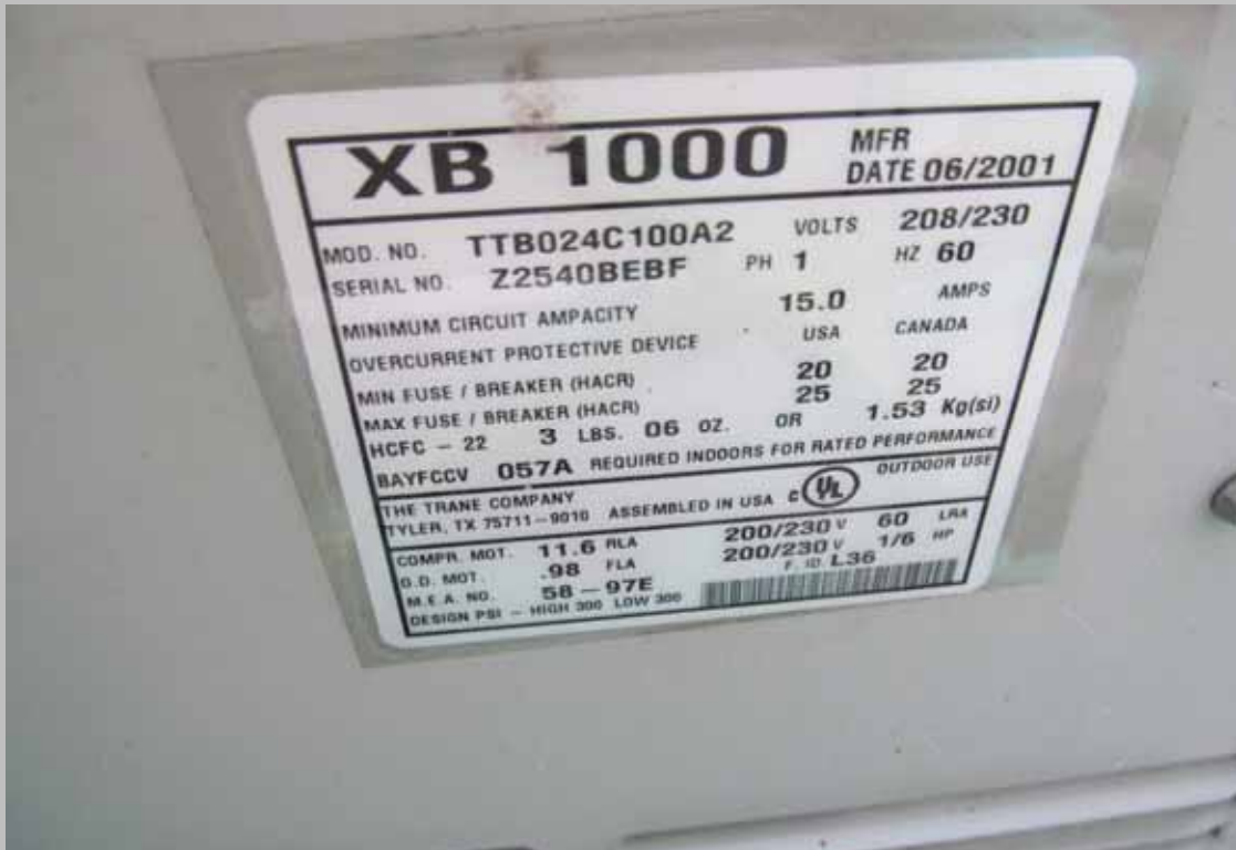
View of typical dwelling unit exterior condensing unit specification tag.
