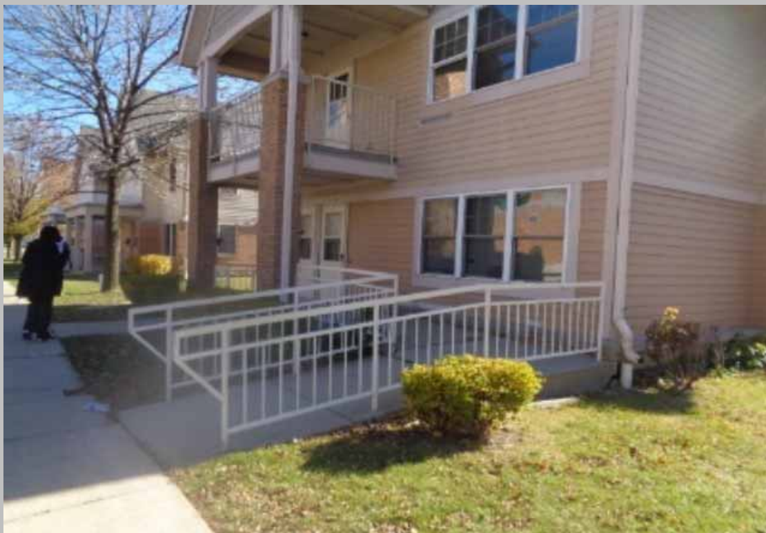
View of typical entry ramp / accessible route to ground floor units.
