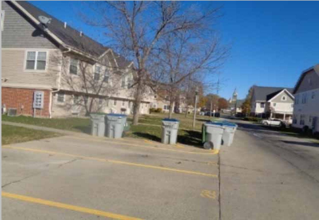
View of typical concrete driveway and parking areas.
