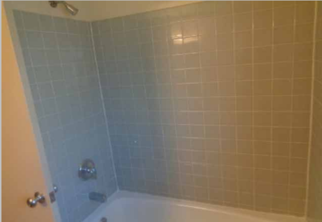
View of typical dwelling unit tub/shower.
