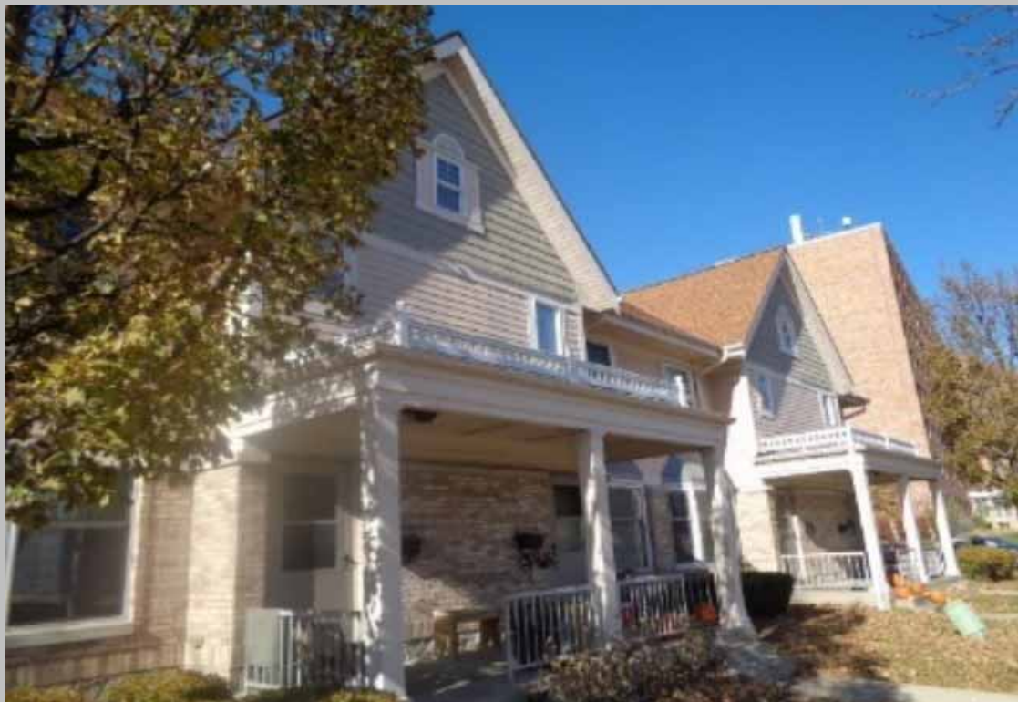
View of typical building elevations at various building types.
