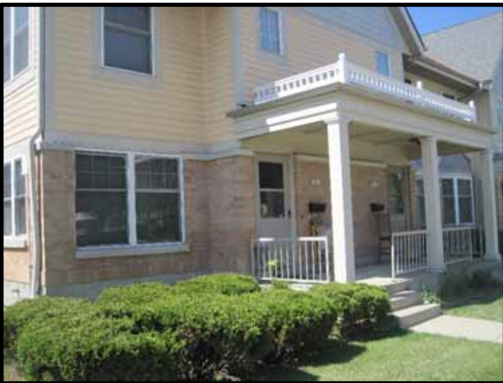
Typical Porch of Subject Building
