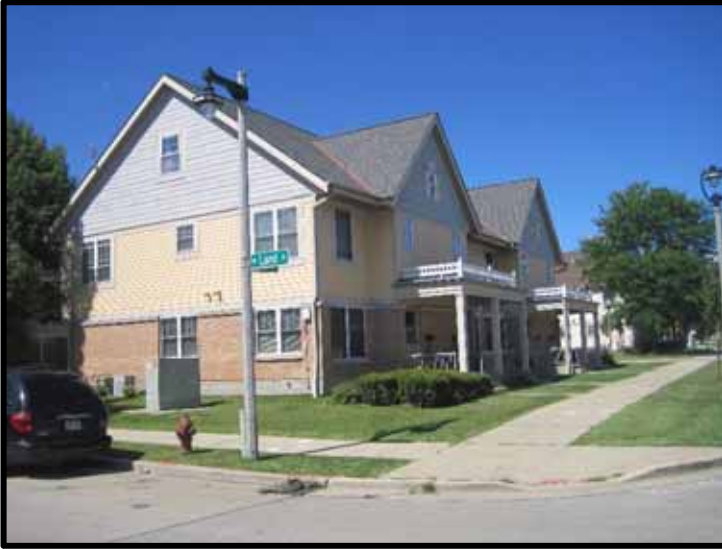
Typical View of Subject Building
