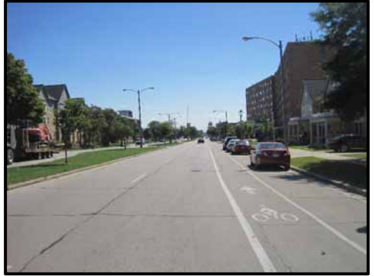
Looking South along North 6 th Street e
