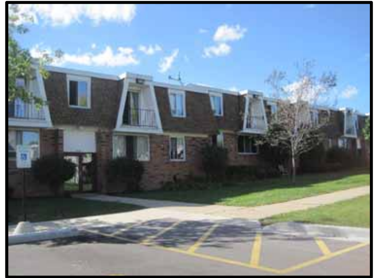
Plymouth Apartments Southwest of the Site
