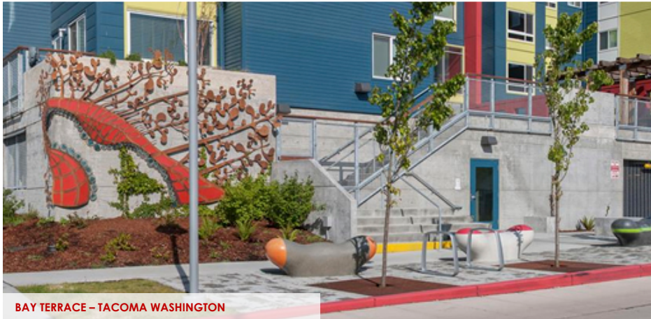
BAY TERRACE – TACOMA WASHINGTON
