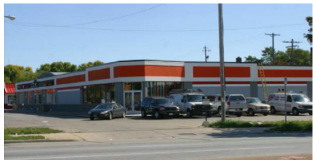
AutoZone's Facade Transformation (HACM)
